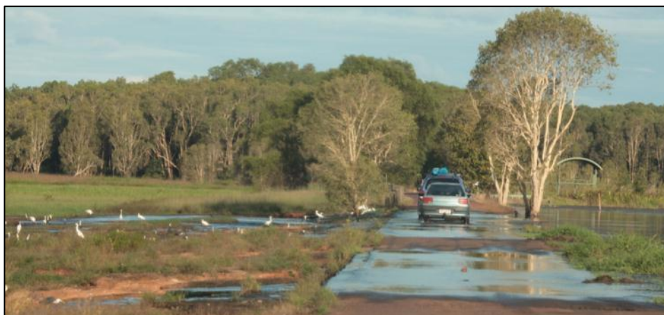
The elevated dam wall at Fogg Dam provides a raised, single-lane sealed road along which visitors can drive (Photo: © Michael J Barritt)
